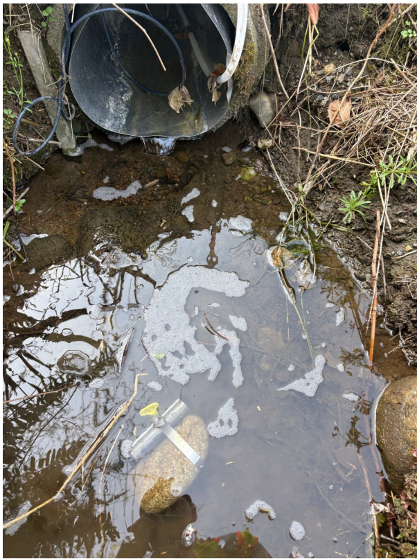
Photo of intake tubing going into pipe.
