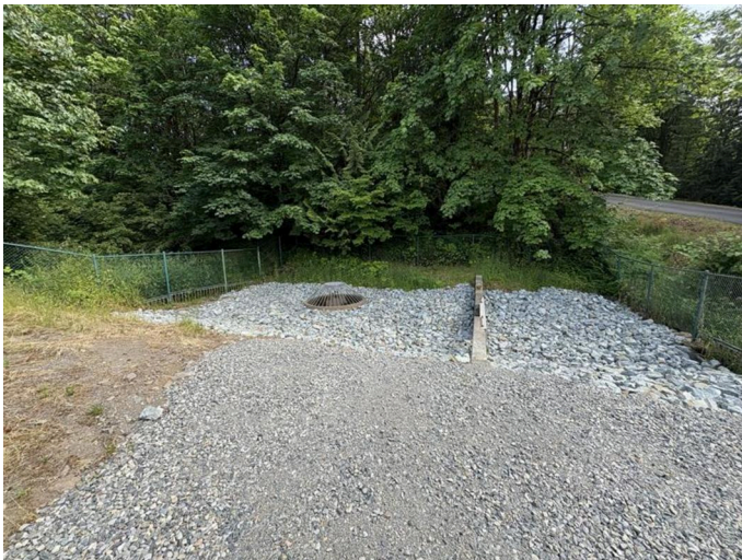
Side view of entire monitoring location. Stream channel covered in riprap
