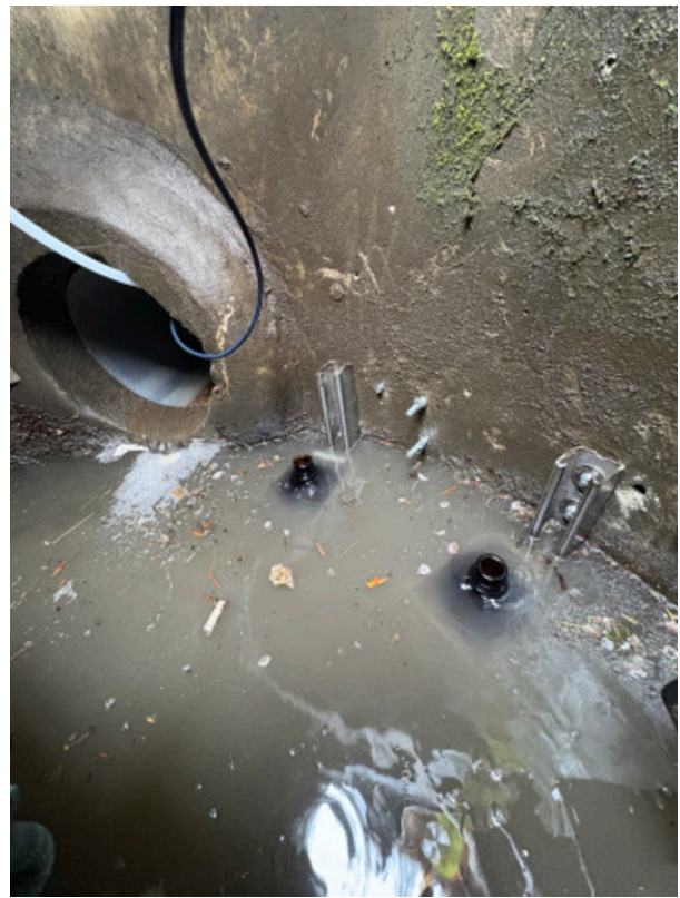
sediment trap position relative to flow meter
