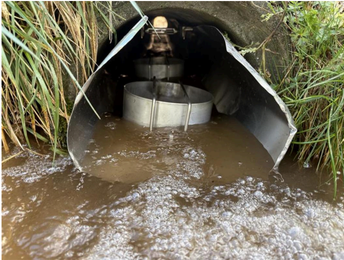
View of sediment traps installed within pipe system
