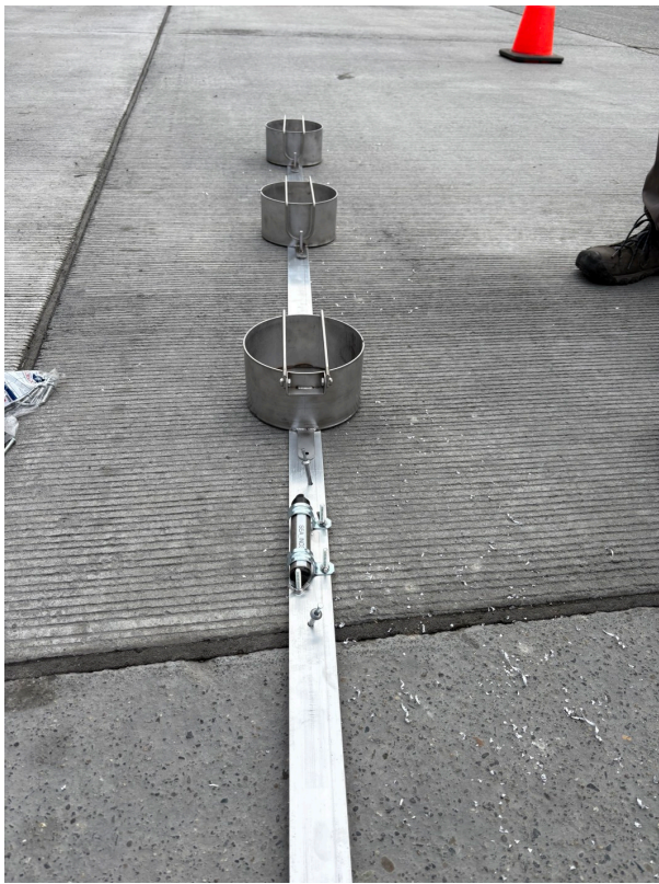
Sediment traps prior to installation
