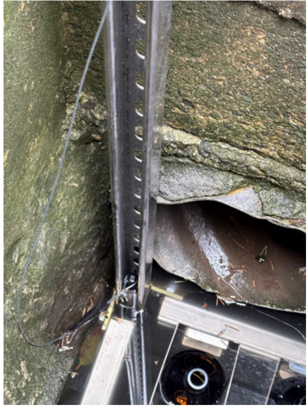
Pressure Transducer location inside CB
