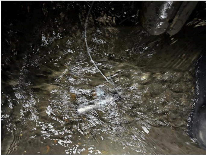
position of pressure transducer at the site (underwater).
