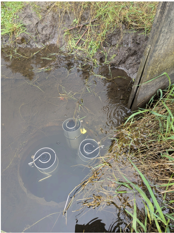
close-up view of sediment trap installation
