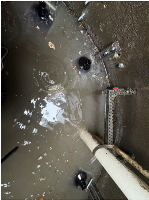
Bird-eye view of all 3 sediment traps inside the sump
