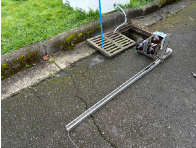
Full view of sediment trap equipment before install
