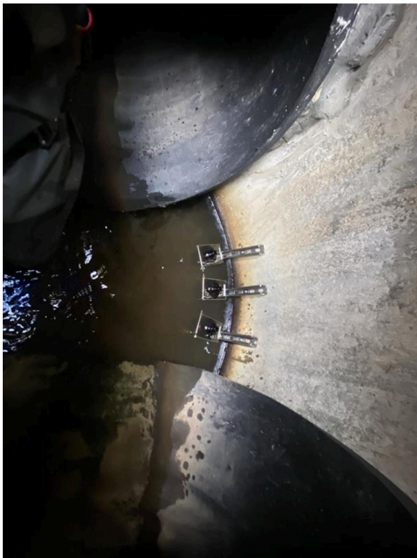
Bird-eye view of sediment trap location within pipe
