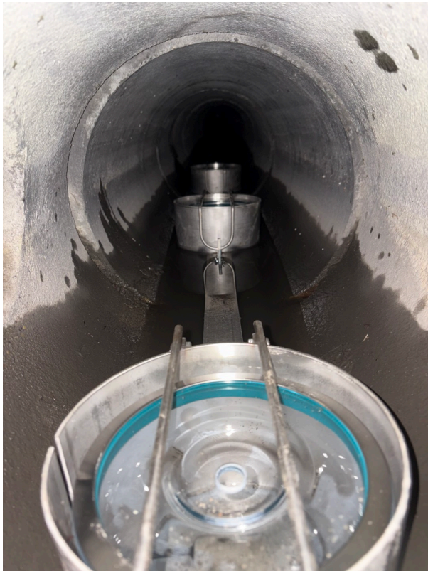
close-up of sediment trap inside pipe
