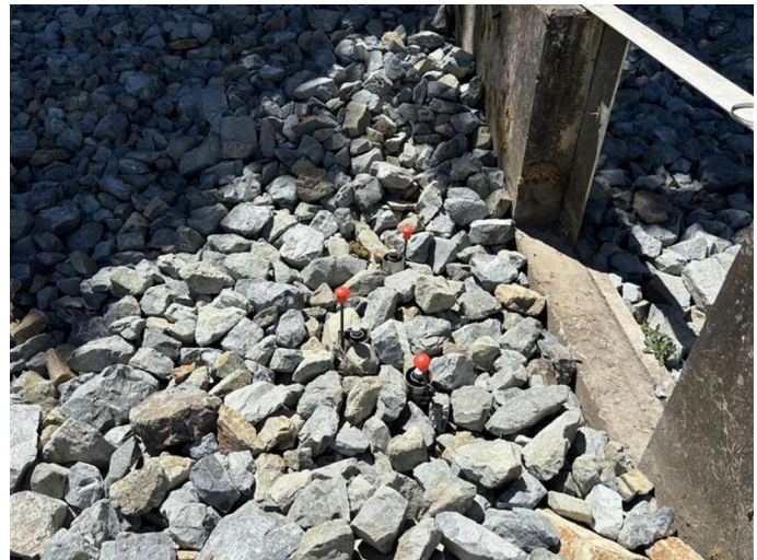
Sediment traps (red markers) installed just downstream of weir structure along width of the channel
