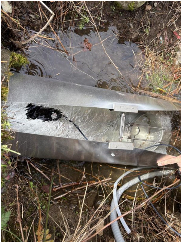
Flow sensor in sheet metal, expansion clamp set-up prior to installation in pipe. Flowmeter installed in downstream portion of pipe, just before outlet, N side of driveway
