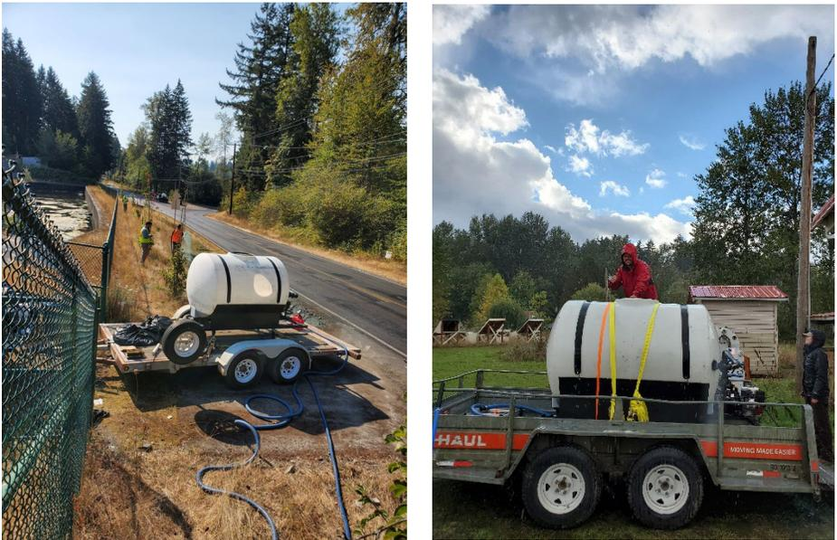
Figure 5: Hydroseeder used to spread plant seed.
