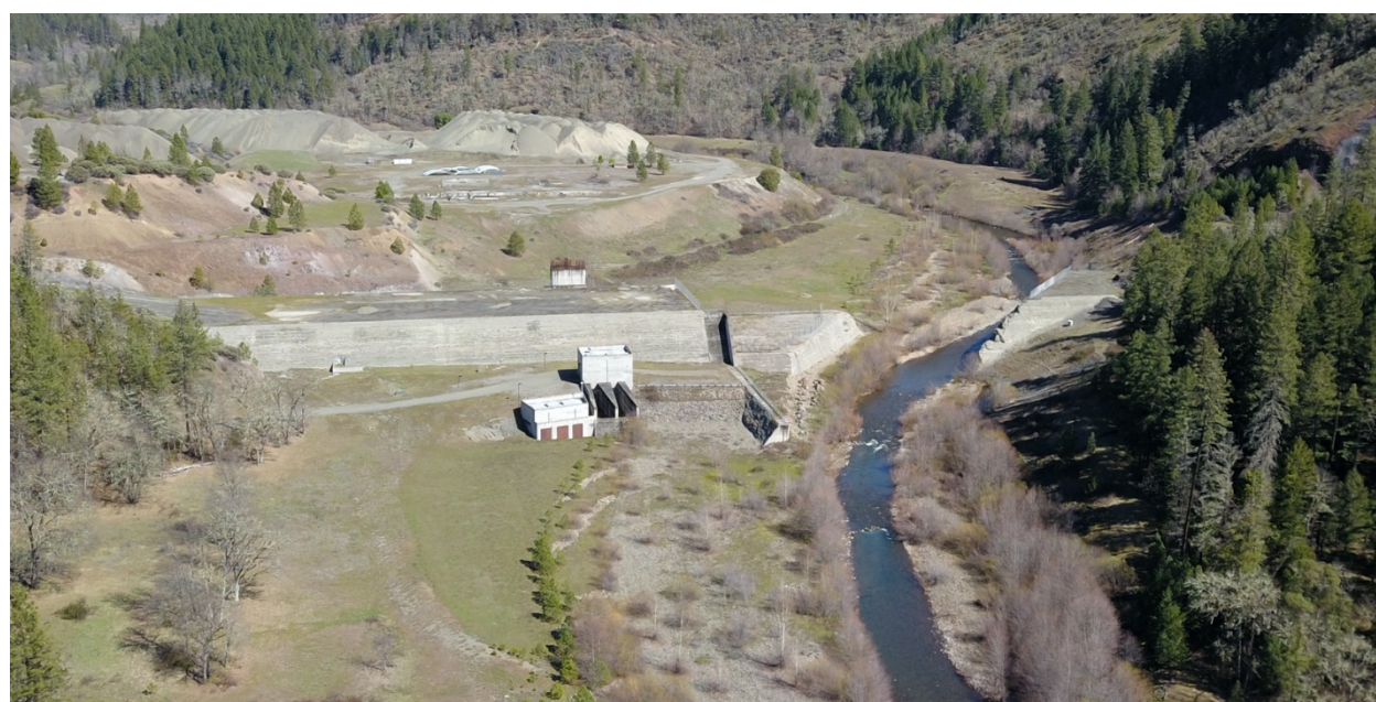
Figure 8 Looking Upstream at Elk Creek Dam (View shows partial removal to allow Elk Creek to freely flow through the roller compacted concrete structure.)
