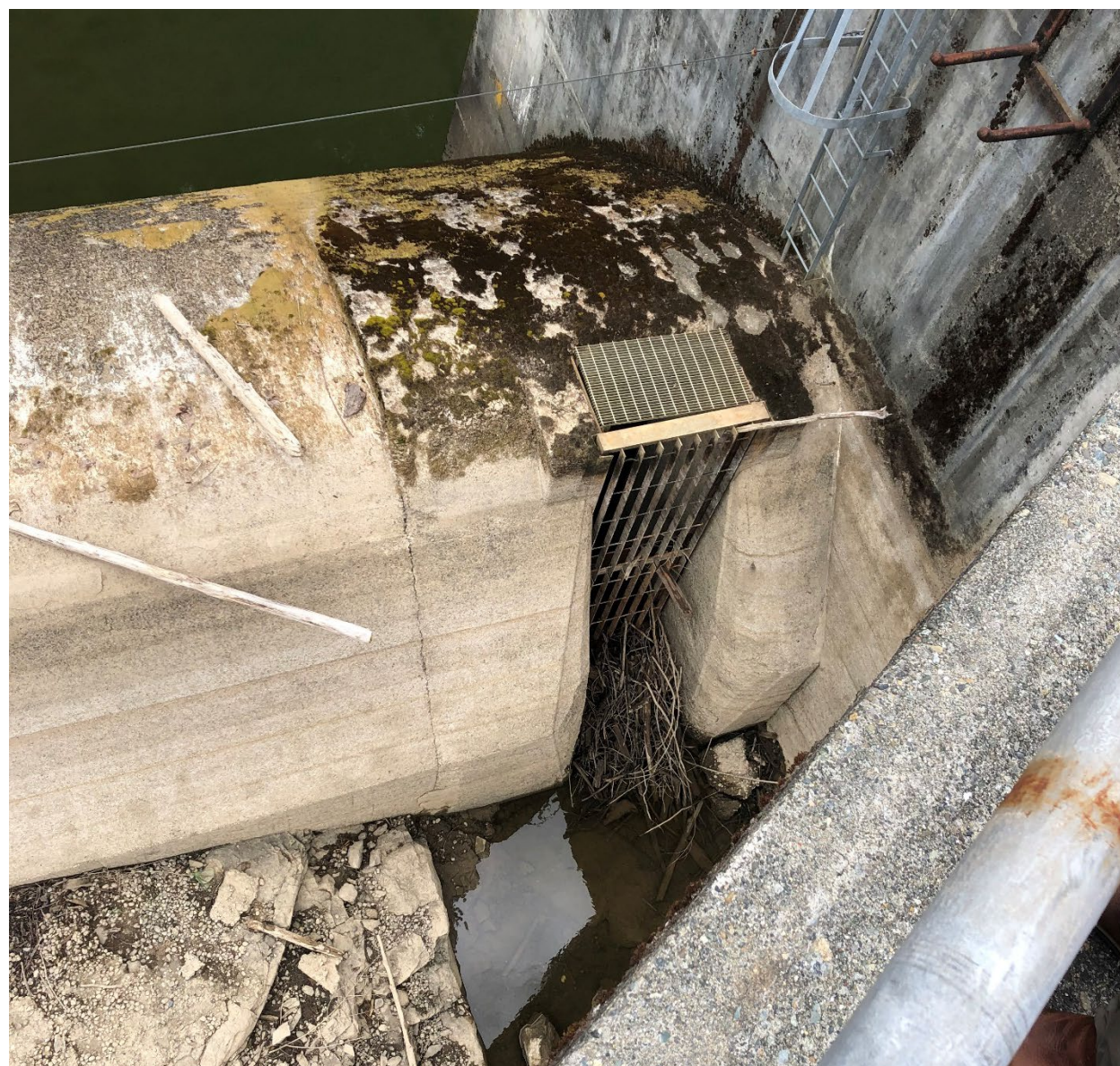
Figure 3 Photograph of Fish Sluice in Spillway
