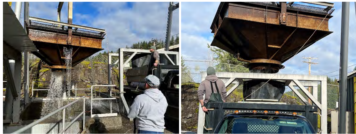
Figure 4 Transport Truck Loading Hopper and Hoist
