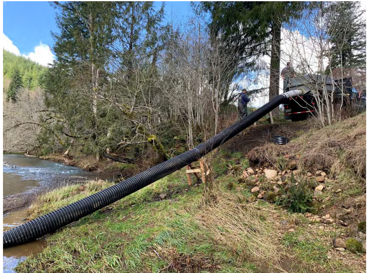
Figure 7 Current Truck Release Hose
