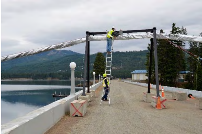
Fig. 5. Simple over-road tube hanging structure
