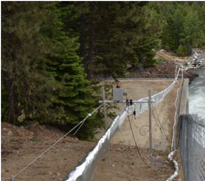
Fig 3. Simple support stand for over land tube section
