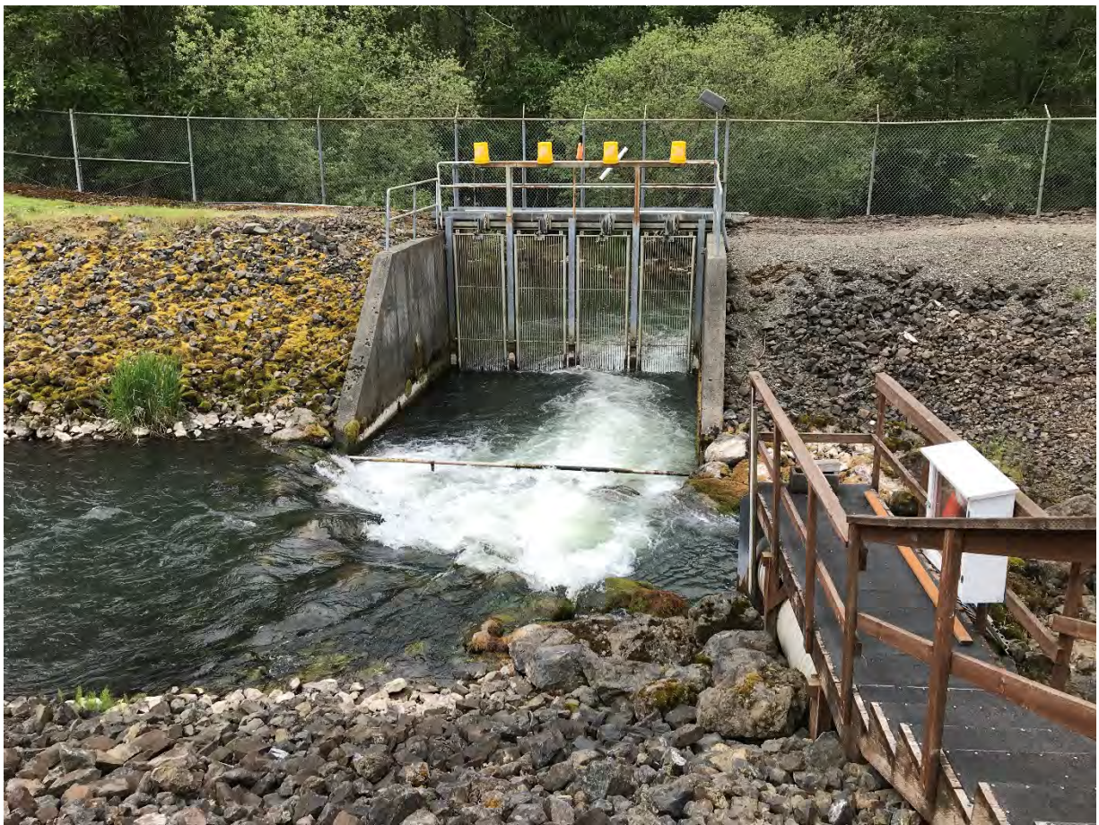
Figure 2 Rearing Pond Exclusion Barrier
