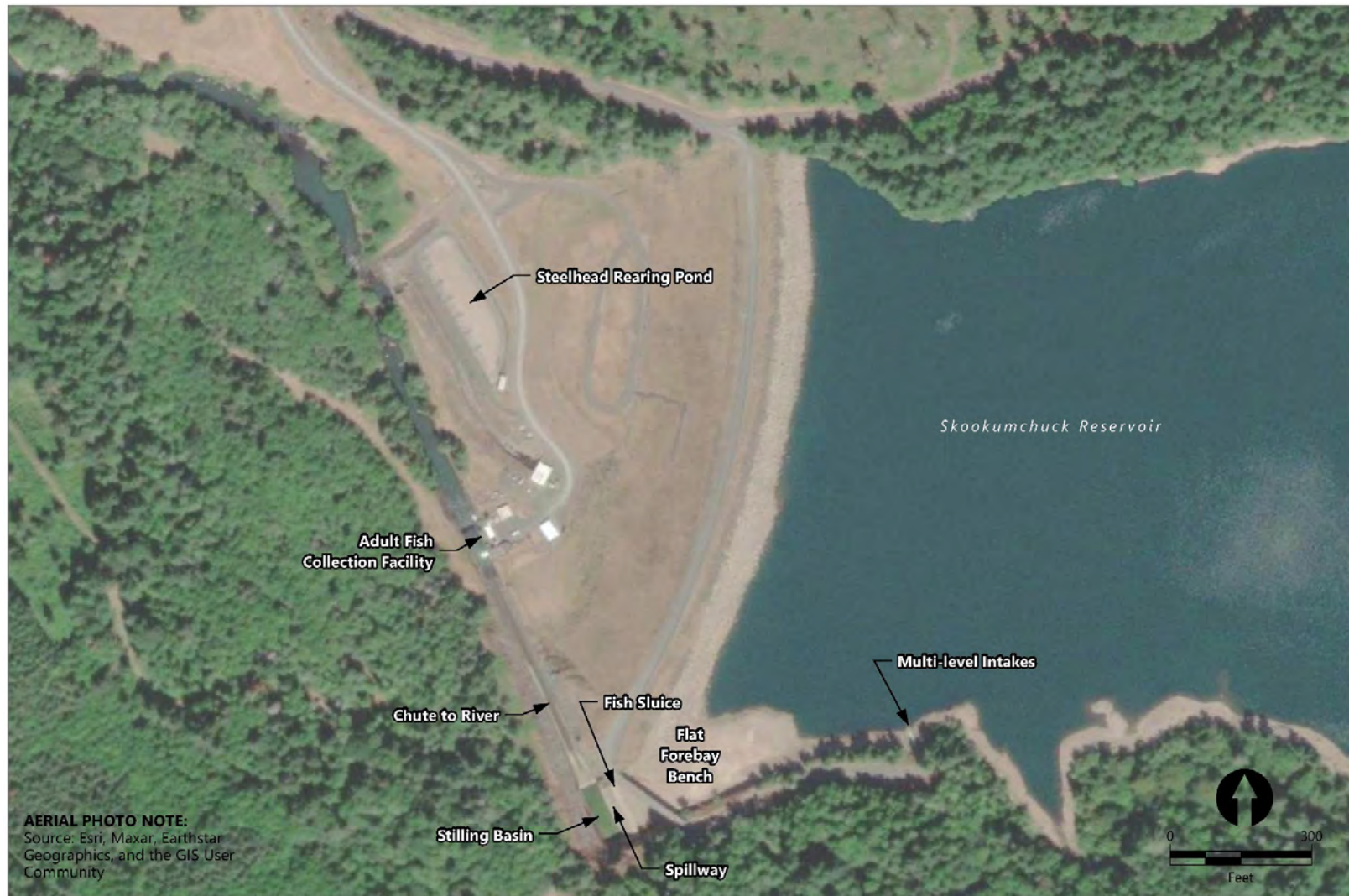
Figure 1 Major Site Features of Skookumchuck Dam
