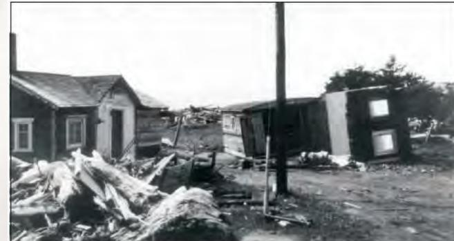
**Figure 5.** Photo 8-2-A. Portion of house completely torn from main part. Entire house was moved northwest 40 ft (12.2 m) from foundation. Map location 9.
