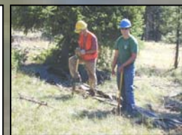
Installing silt fence
