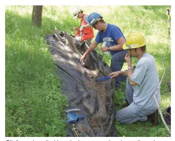
Silt fence installed lengthwise across the slope allowed scientists to collect and measure the amount of eroded materials.
