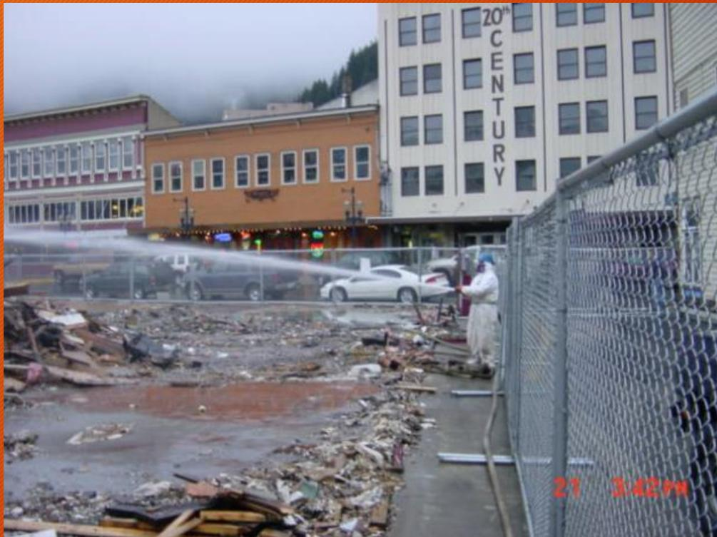
Abatement workers apply water before, during and after removing asbestos.
