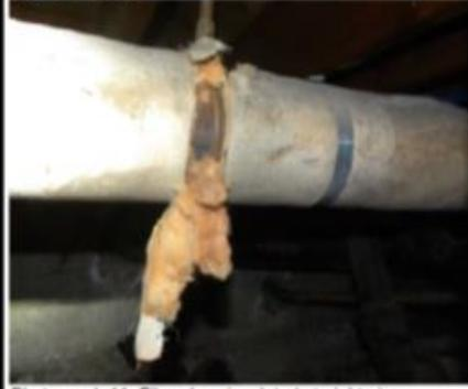
Photograph 11: Fiberglass insulated straight pipe insulation on crawlspace steam pipes.
