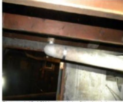
Photograph 12: ACM hard mud pipe fitting insulation on fiberglass insulated pipes in crawlspace.
