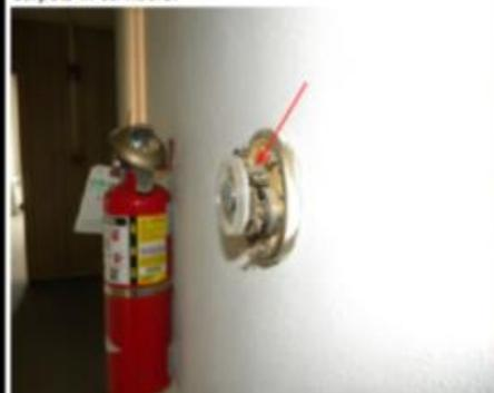
Photograph 5: Mercury switch in lunchroom thermostat.
