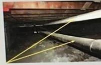
Asbestos pipe insulation in crawlspace
