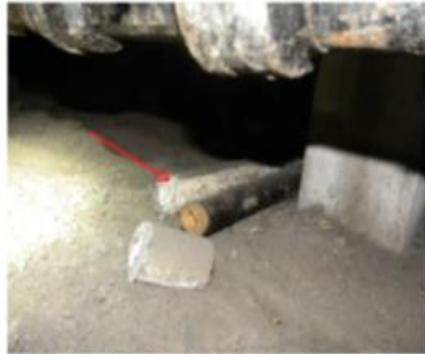
Photograph 10: ACM hot water pipe insulation debris on crawlspace floor.
