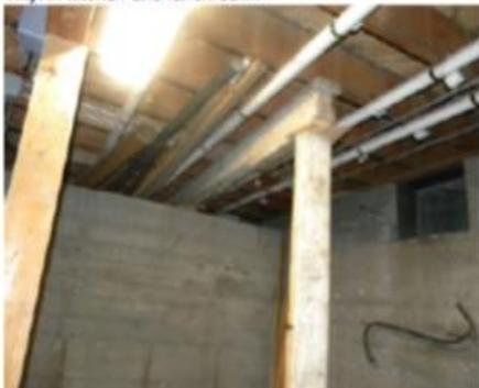
Photograph 6: ACM Aerocel pipe insulation in lunchroom basement.
