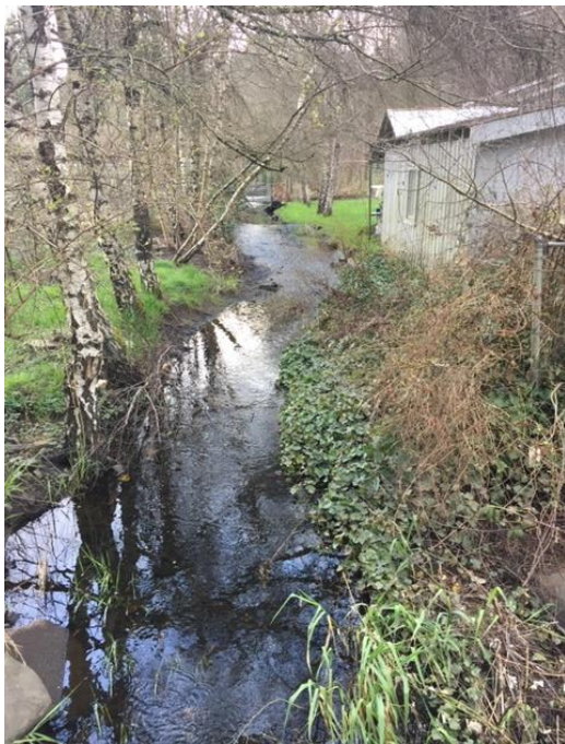
Photograph 4. Riparian intrusion from residential structure just upstream from Site 2 (photograph taken March 25, 2020)
