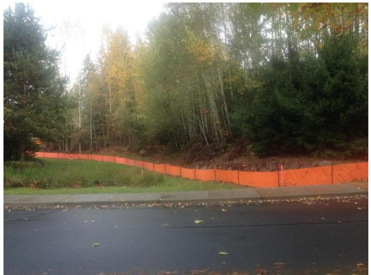
Figure 10. Silt fencing at construction site.
