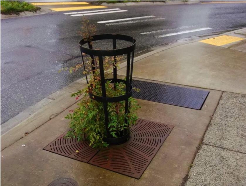
Figure 7. Filterra® system installed along high-traffic roadway.
