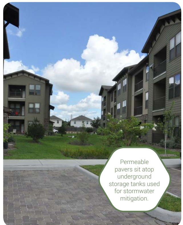
Permeable Pavers and Underground Storage Tank, Queenston Manor
