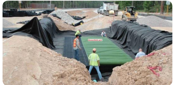
Bioswale and Underground Storage Construction, Birnamwood Drive
