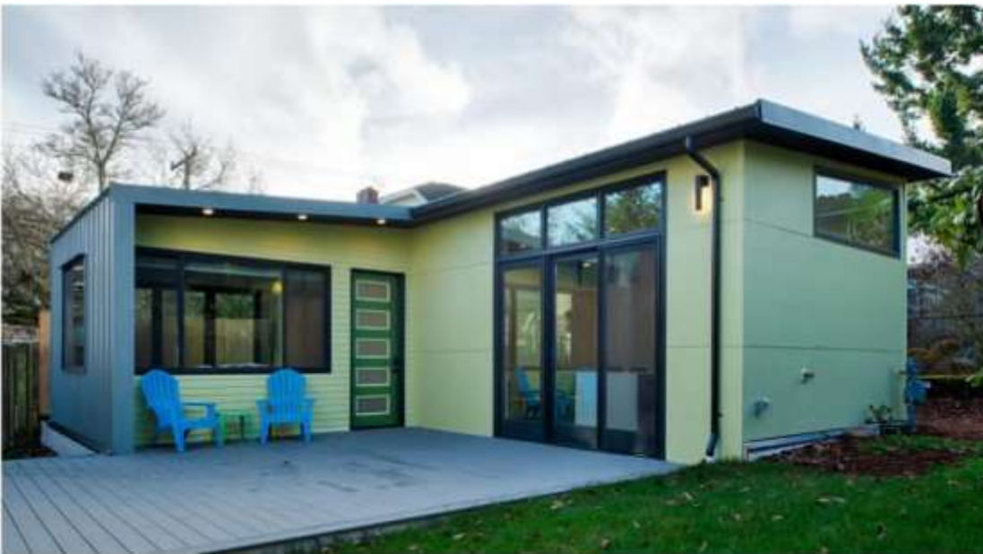
Smith Gillman Cottage converted garage. Credit: CAST architecture.
