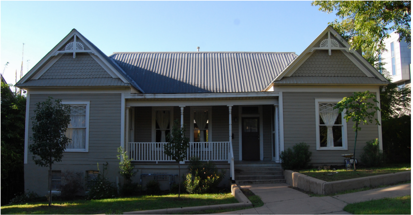
Example of an Engaged Porch
