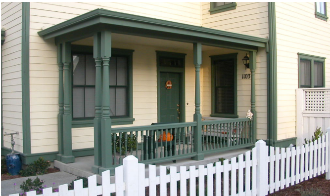
Example of an Engaged Porch
