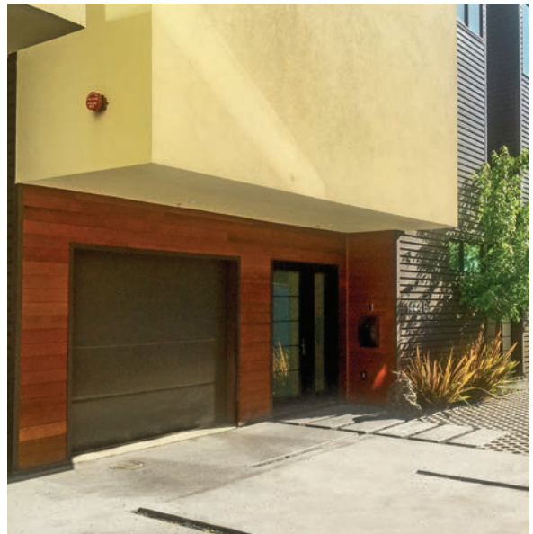
▲ Accommodating cars by adding a garage for apartment residents often lifts a building an additional story, which precludes having active, community-focused spaces on the ground floor.
