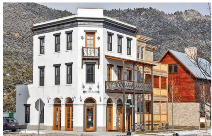
▲ The top two floors of this live/work building in Buena Vista, Colorado, contain a 1,400-square-foot residence. The ground floor can house a shop, office or apartment.
