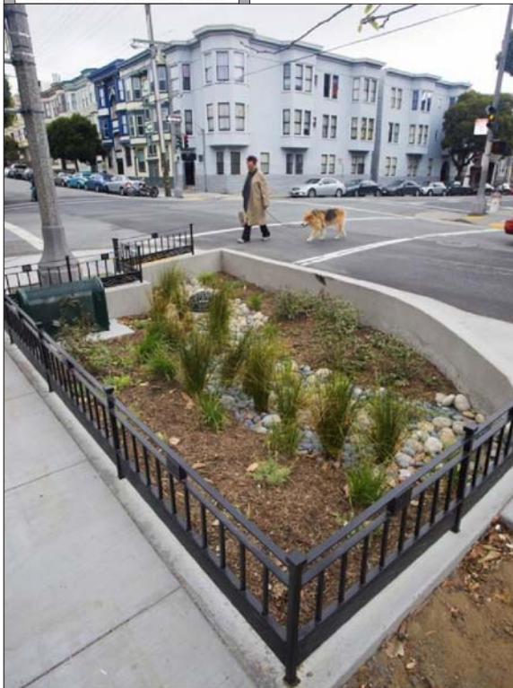
Low Impact Development (LID) projects encourage infiltration, reduce surface water runoff, and promote groundwater recharge.
