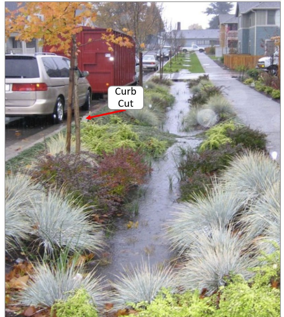
Bioswale Longfellow Creek Watershed West Seattle, WA
