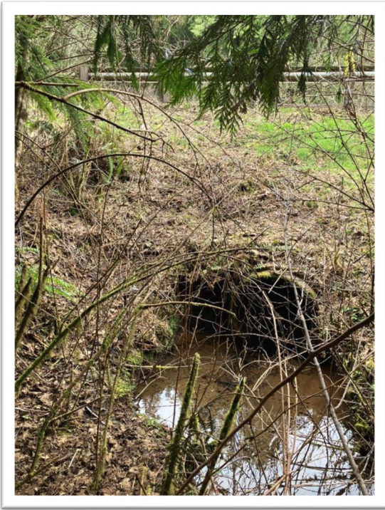
Before – 3-ft pipe
