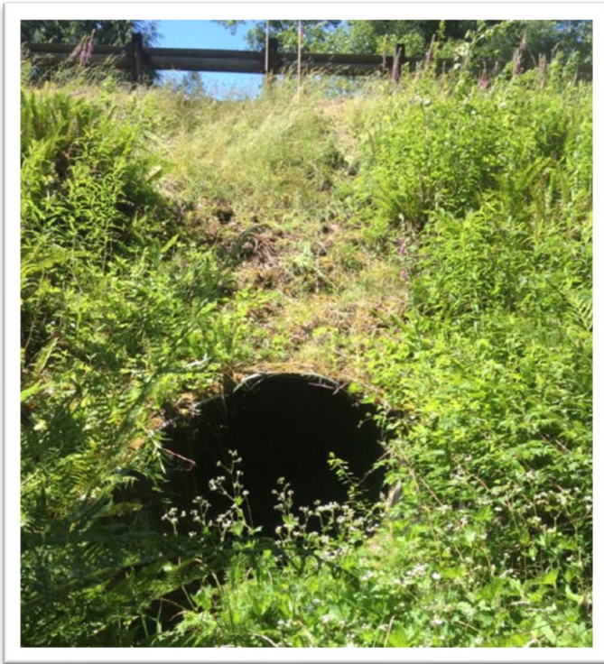
Before – 4-ft pipe
