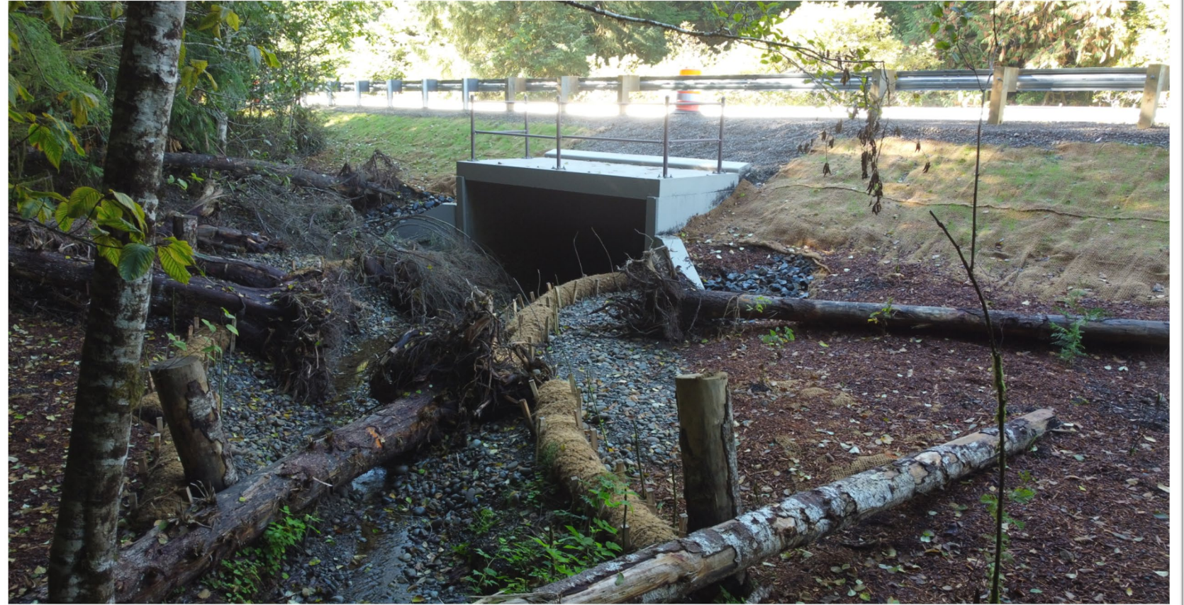
After – 13-ft box
