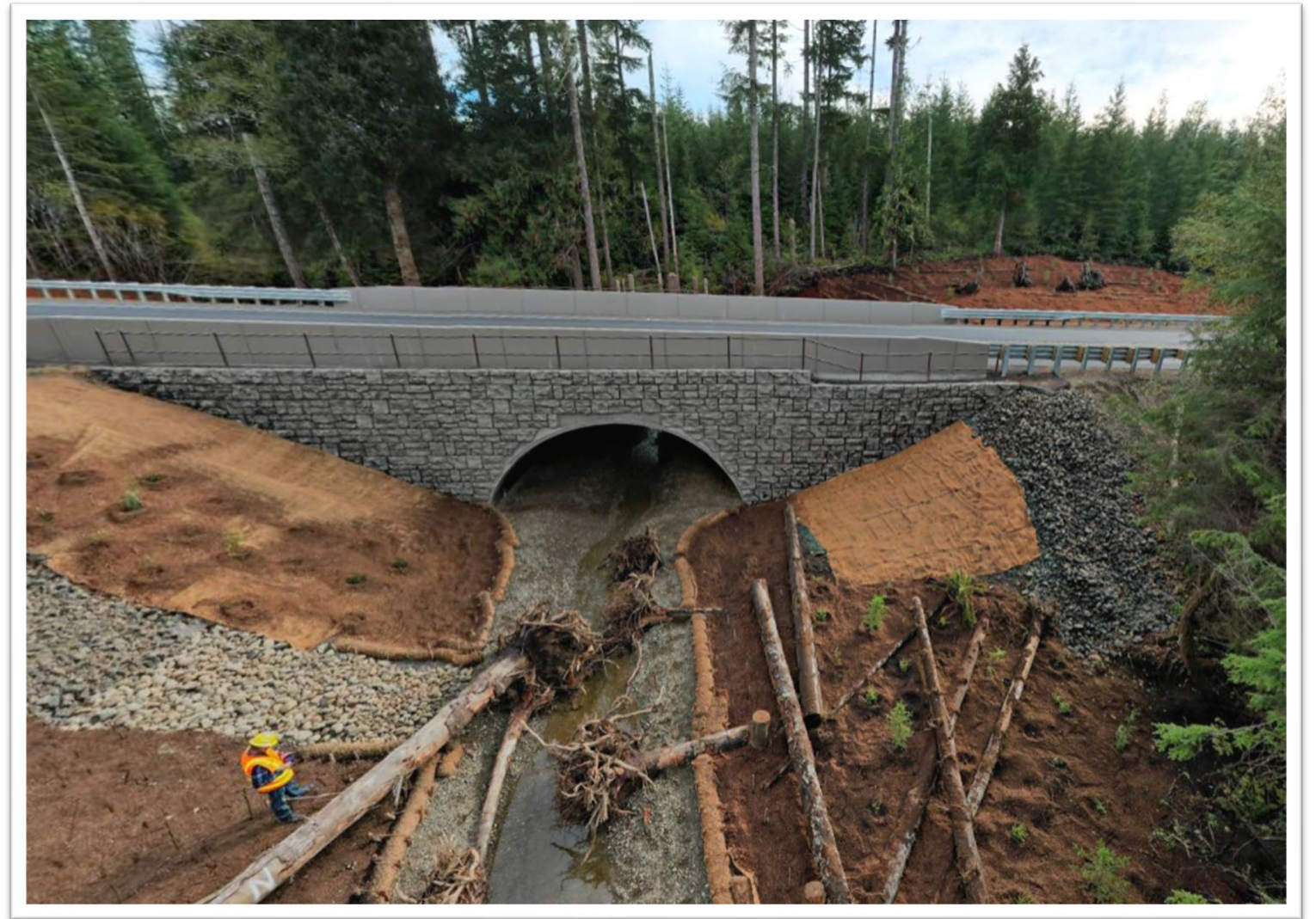
After – 28-ft arch
